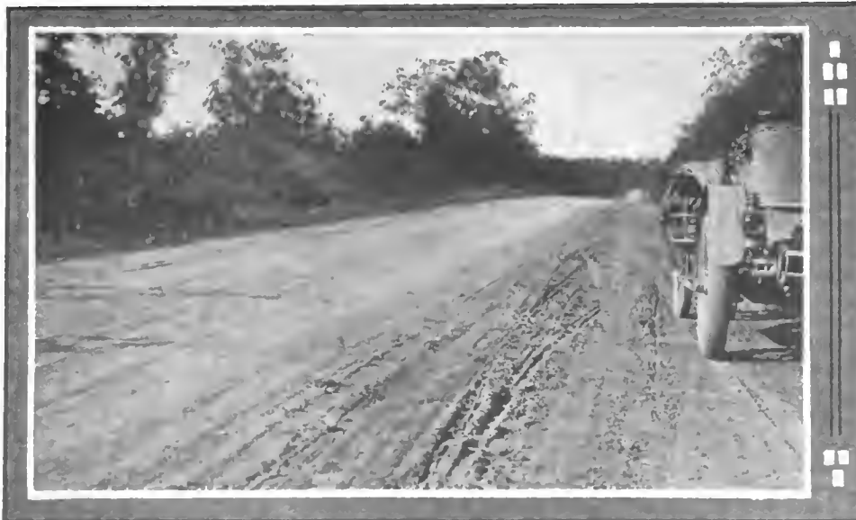
New Jersey Road with Clay Road Bed Surface—Fairly Satisfactory
